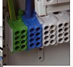
The fitting of terminal blocks\* aids the connection between power supply lines
